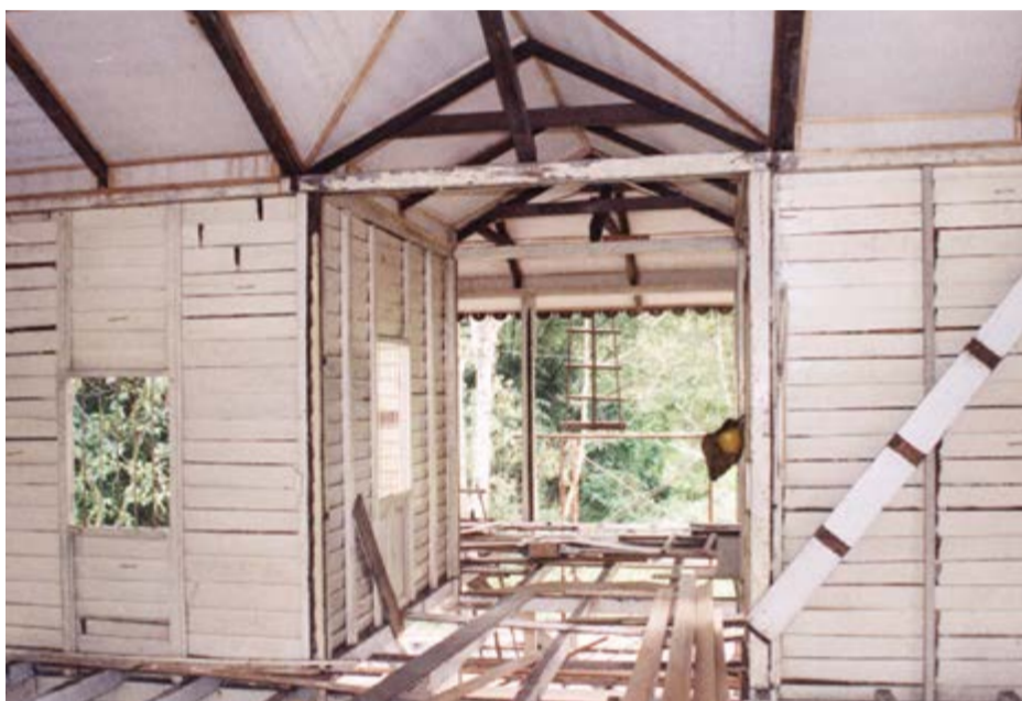
Internal reconstruction involve installing a new timber planks as flooring
