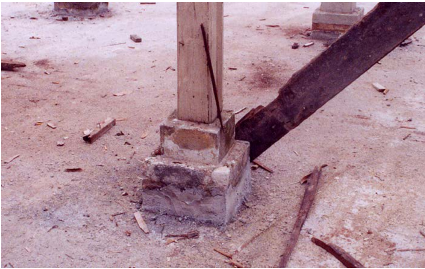
After the completion of the foundation works, the next stage is erecting the timber columns into their respective place
