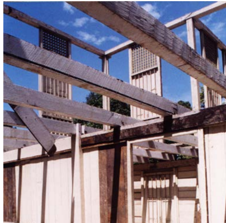
Details of the timber joint and the lattice work at the anjung
