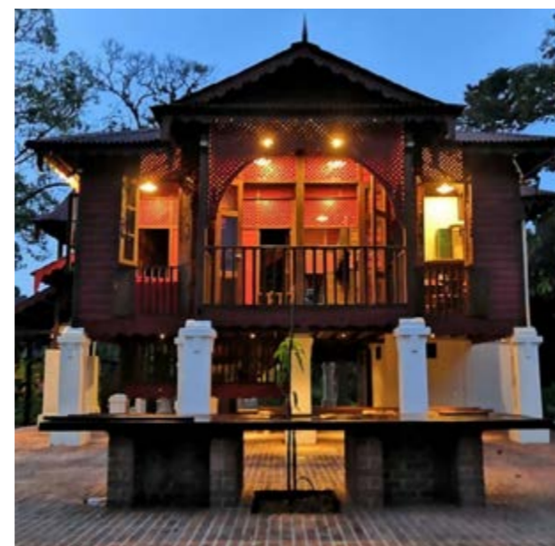
Construction of a Malay Traditional house at Bagas Zakariah, Gopeng.
