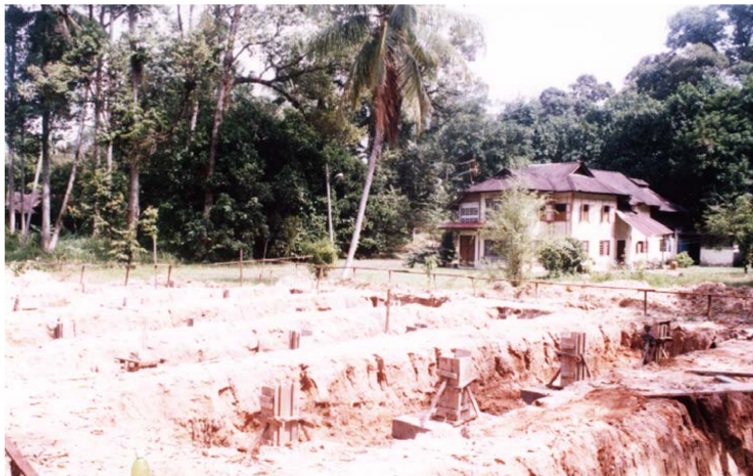
The foundation works starts with R.C footing for the columns
