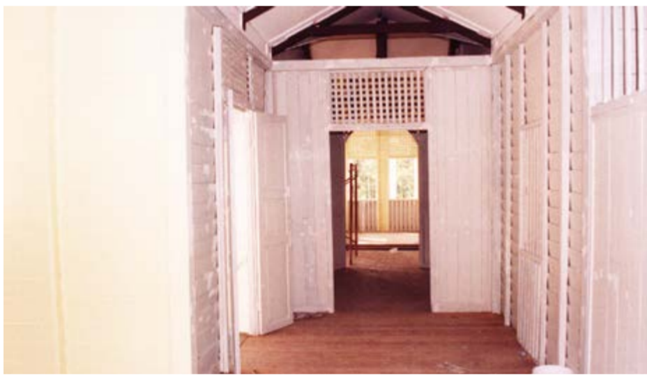
Internal reconstruction involve installing a new timber planks as flooring
