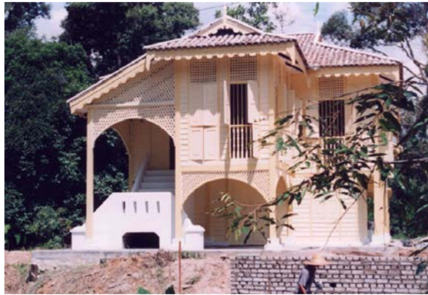
View of the house under restoration.
