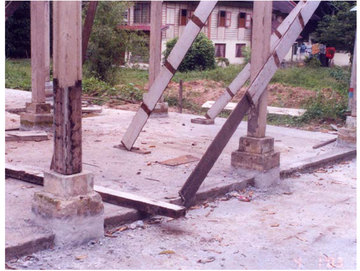
After the completion of the foundation works, the next stage is erecting the timber columns into their respective place
